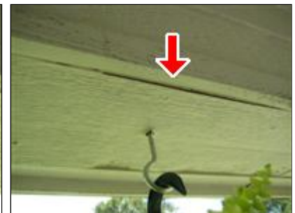
E. Picture 3 SEAM OPENINGS
