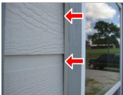
H. Picture 1 OPENINGS AROUND WINDOWS
