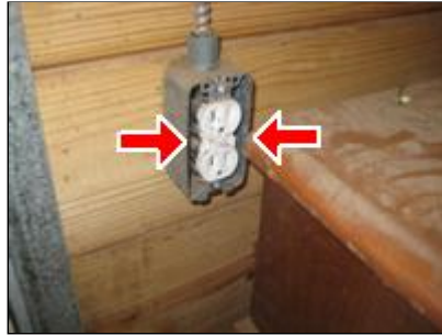
B. Picture 5 Metal garage
