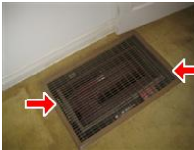
A. Picture 6 FLOOR REGISTER
